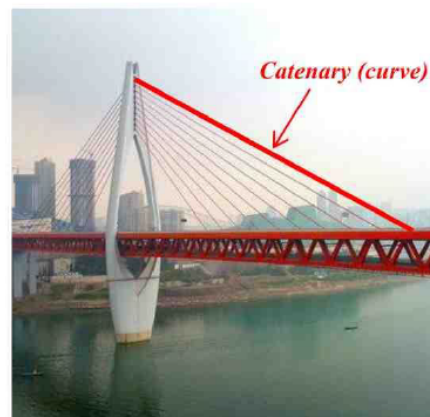
Figure5. Catenary shape in cable stayed bridge.
